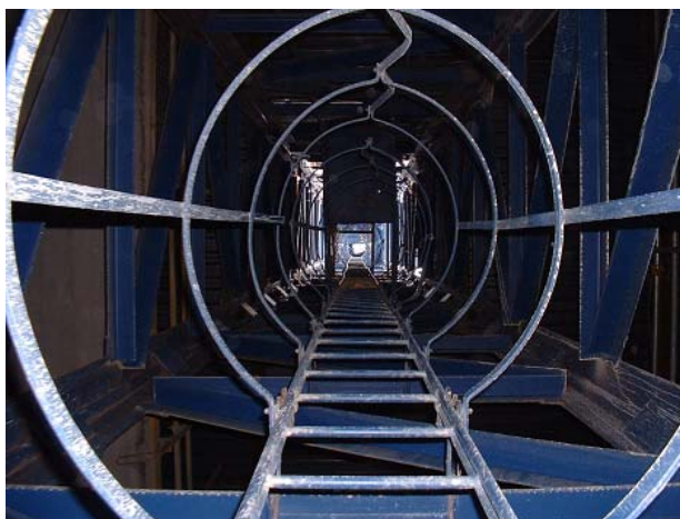
Figure 3 – Single Vertical Ladder
